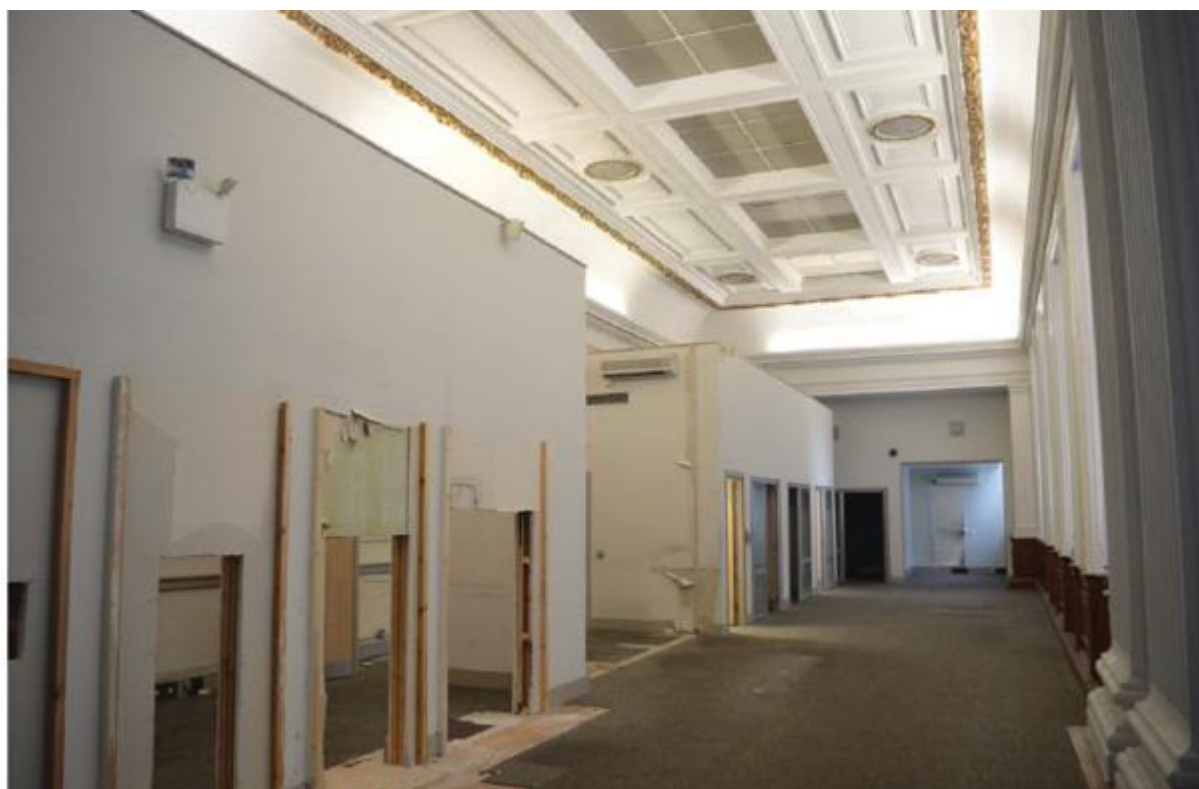
Internal ground floor
